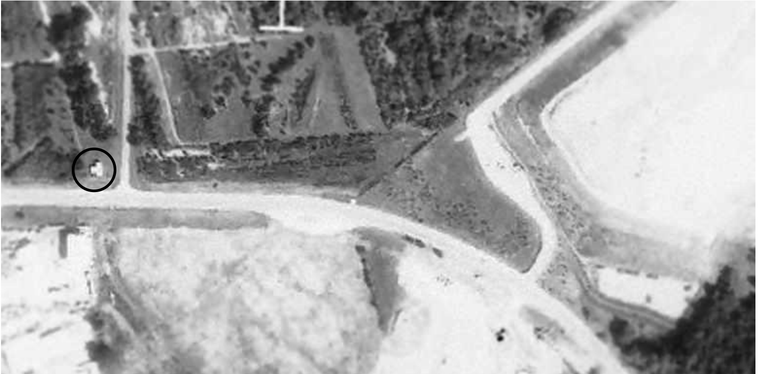
A 1979 aerial photo of the site of Gude Airport (courtesy of Jerry McCauley).
